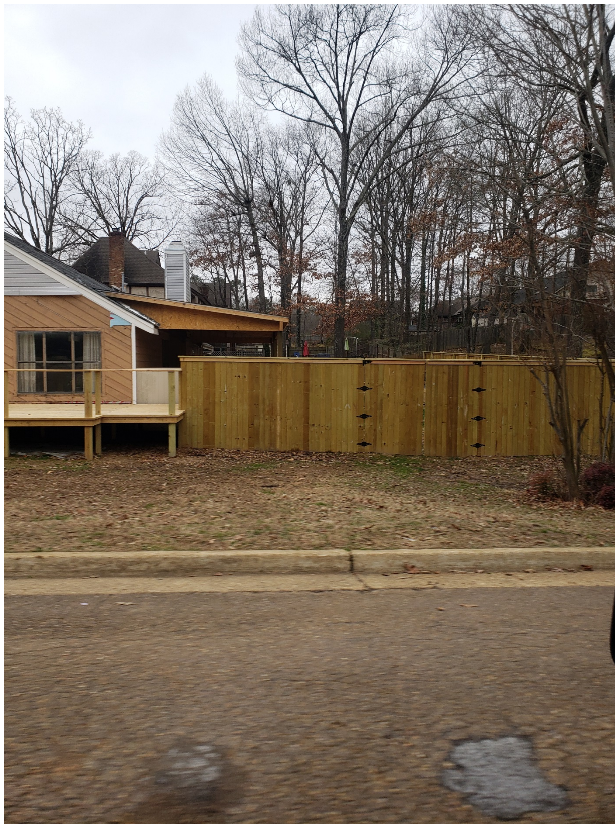
Figure 3: Fence as installed today from Green Spruce Bend.
