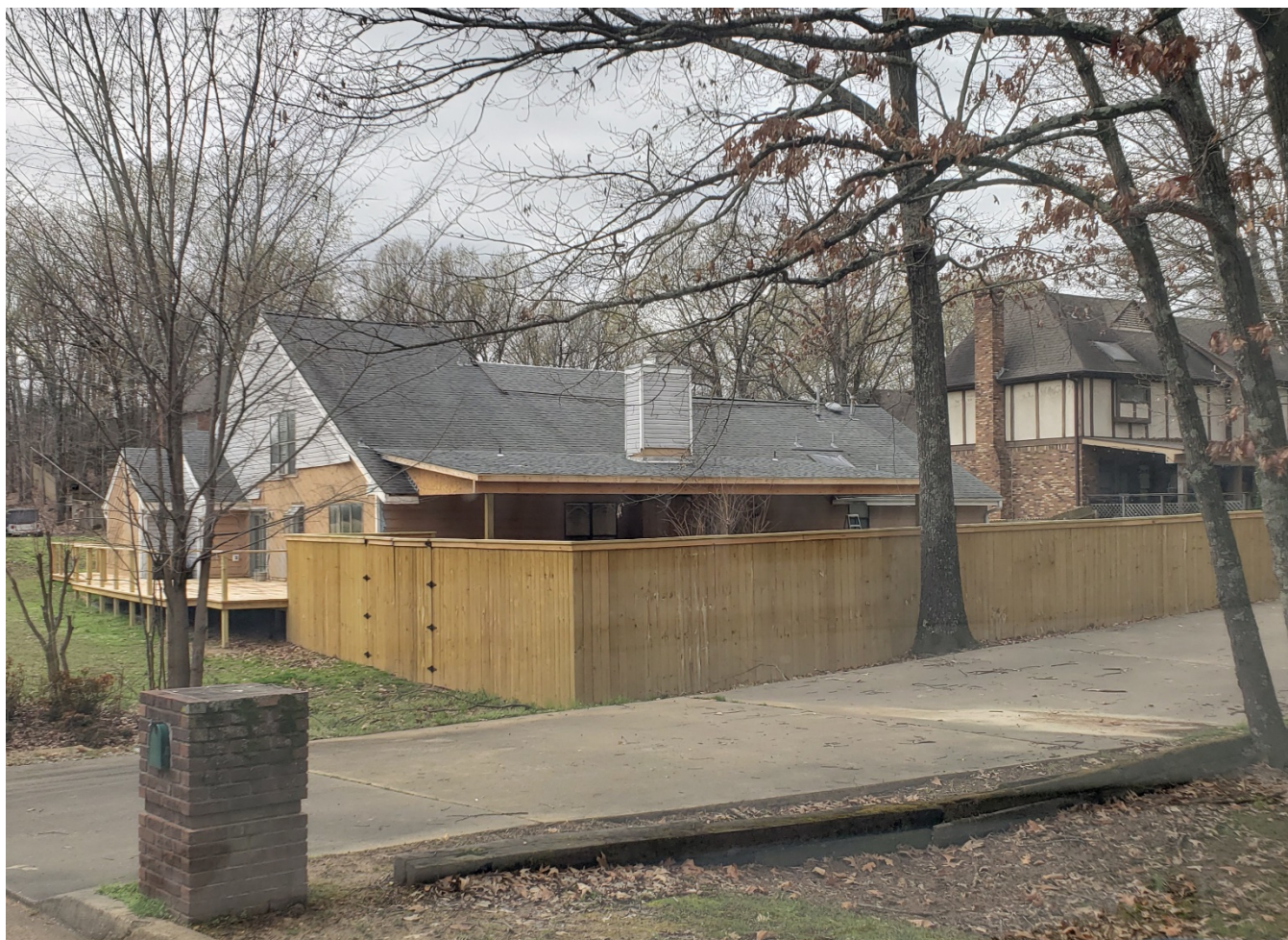
Figure 4: Fence as installed today from the rear property line on Green Spruce Bend.
