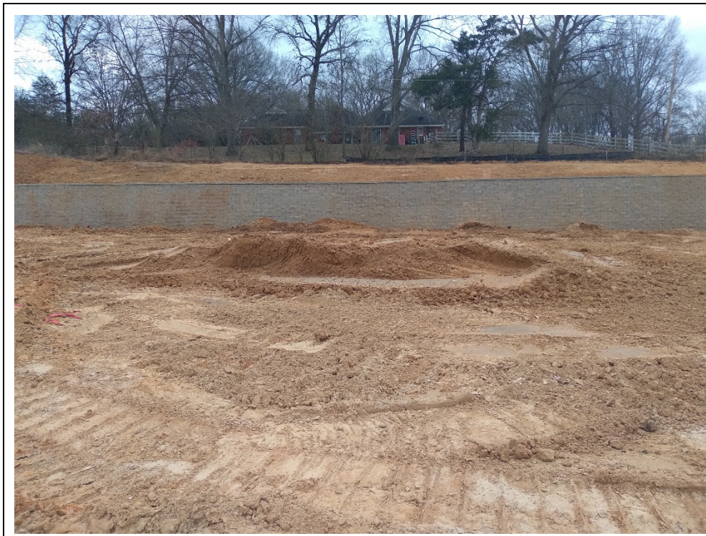
Photo #4: South end of wall #1 with cap blocks installed
