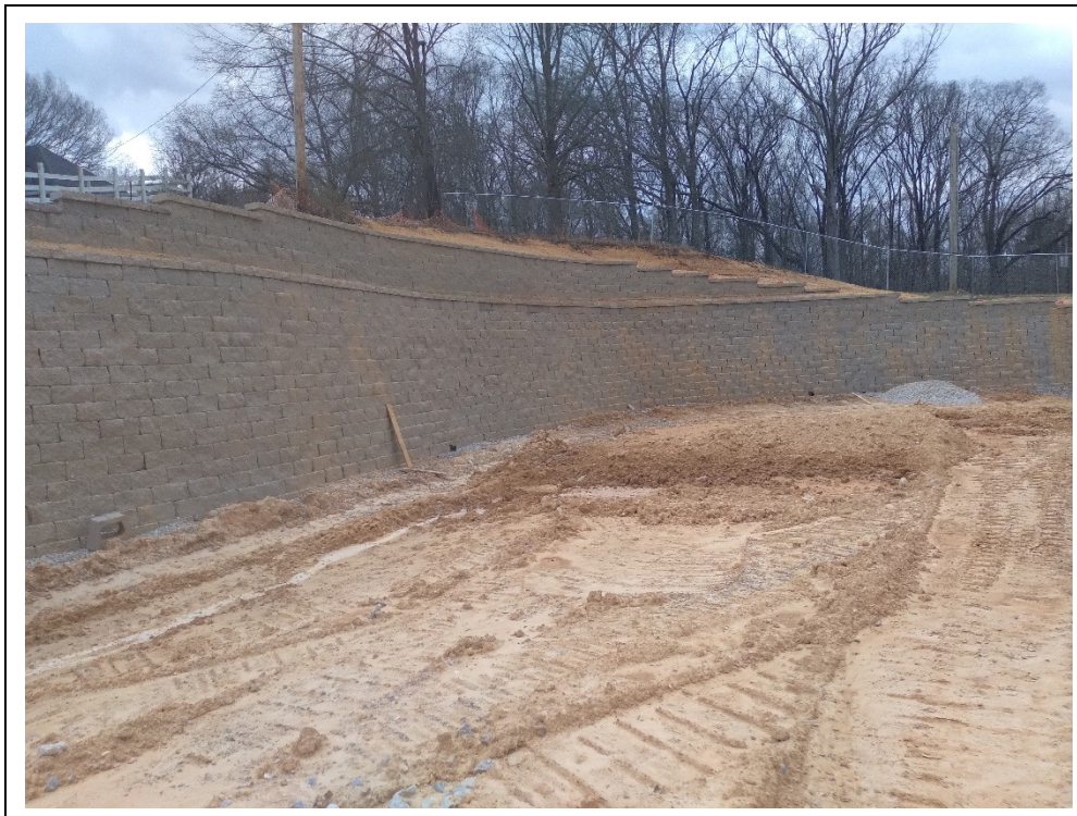
Photo #6: South side wall #1 and #2 looking south
