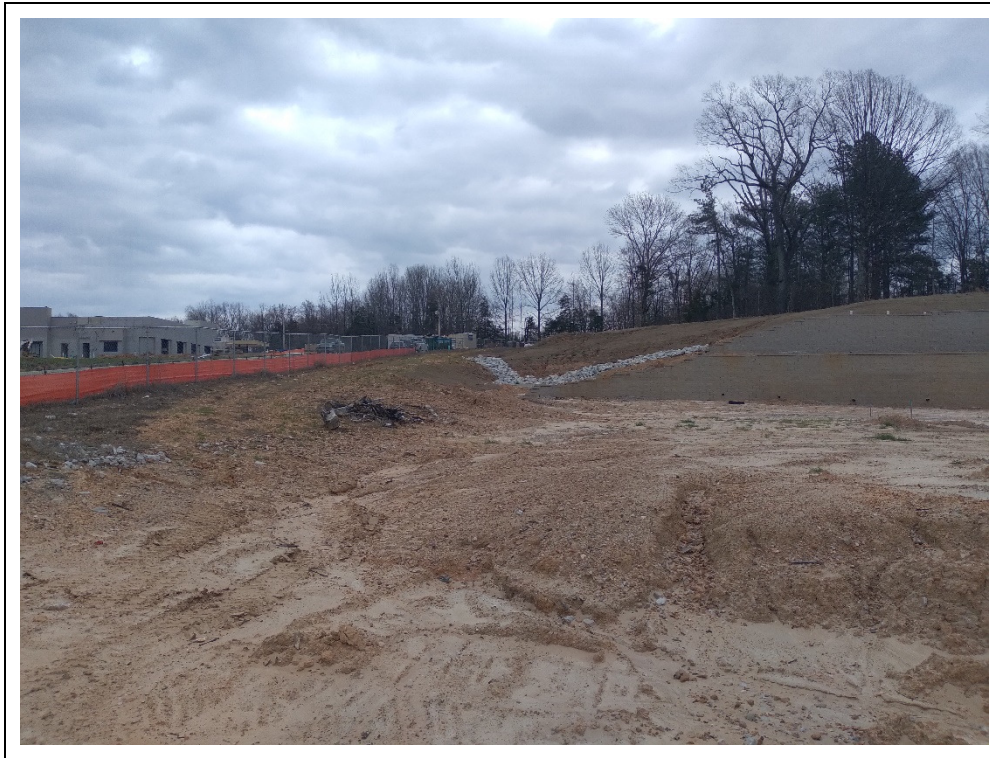
Photo #1: Looking east from entry gate. Wall #1 and #4 are visible.
