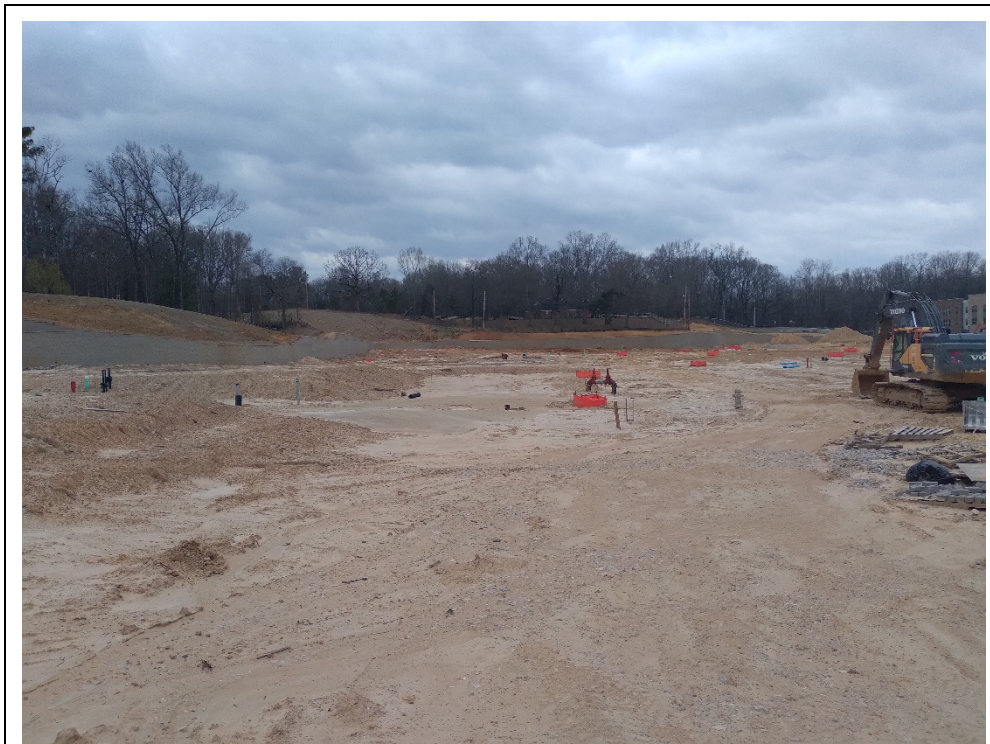
Photo #2: Looking south from Village Market Lane. Temporary inlet protection is in effect.
