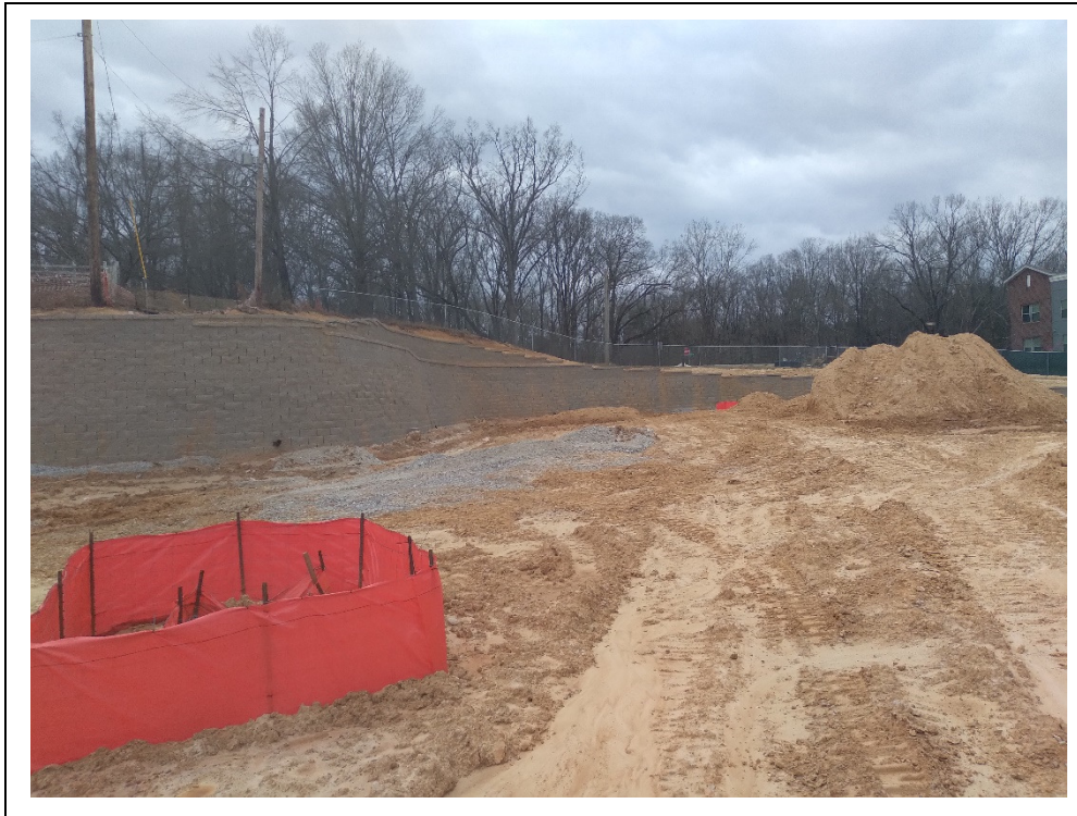
Photo #5: Wall #1 construction is complete. Compacted stone base and geo-fabric have been utilized per details
