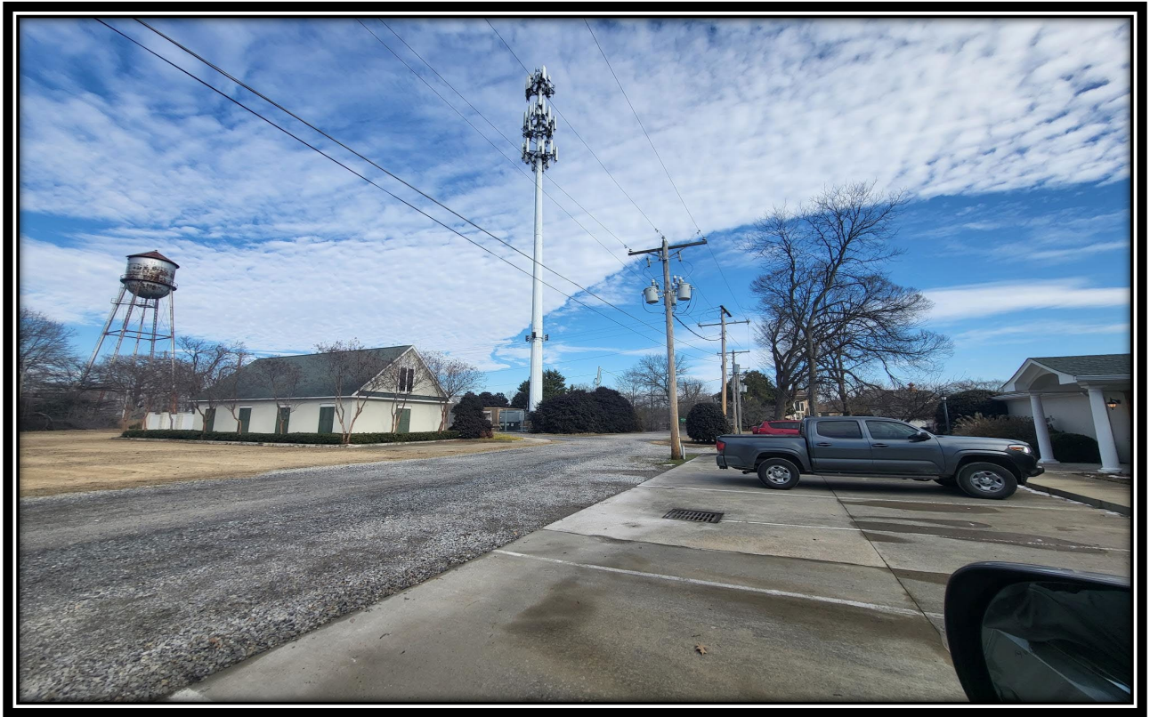
Marion AR –Tower -Site
