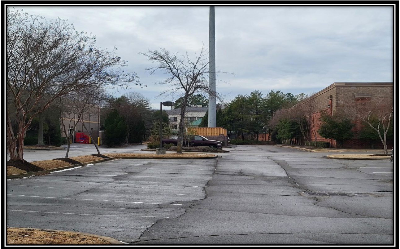
Germantown, TN – OfficeMax – Site
