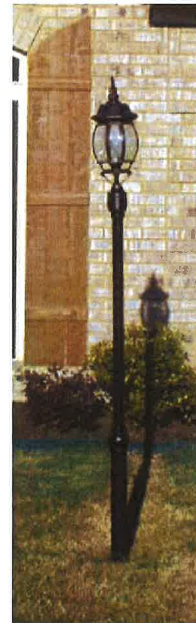
TYPICAL LIGHT - ONE PER EACH FRONT YARD
