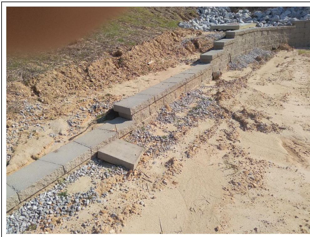
Photo #4: No North end of wall #1 with cap blocks installed
