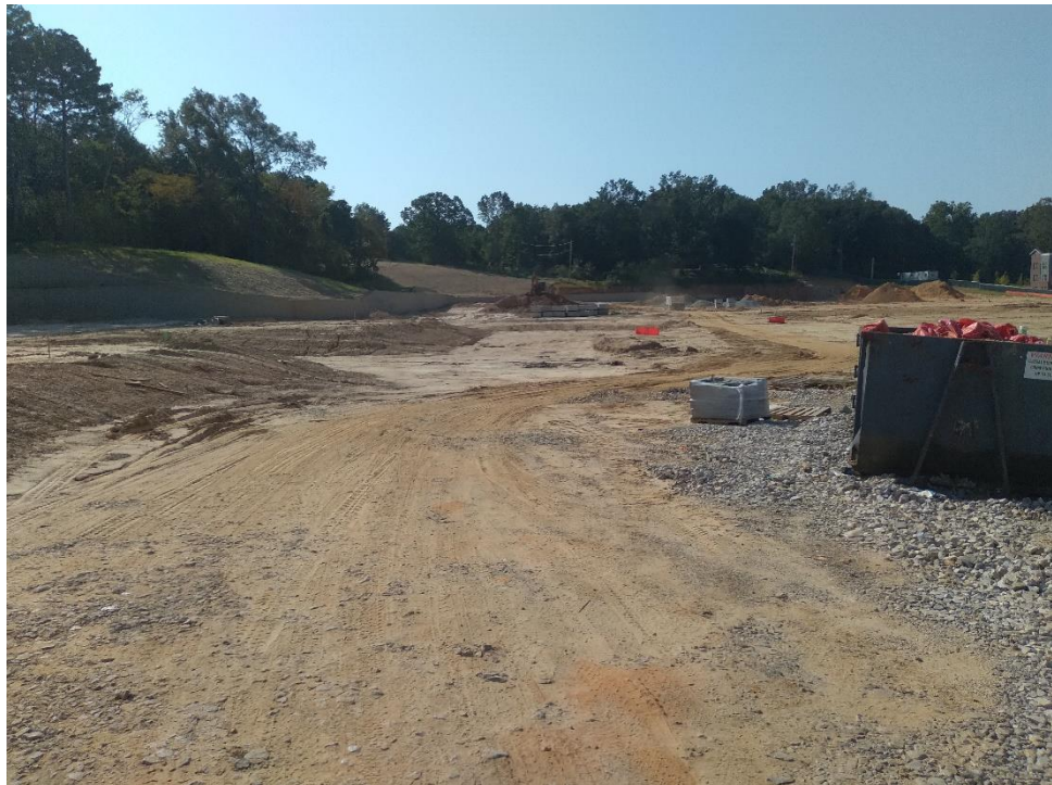
Photo #2: Looking south from Village Market Lane. Underground utilities are complete at the south end.
