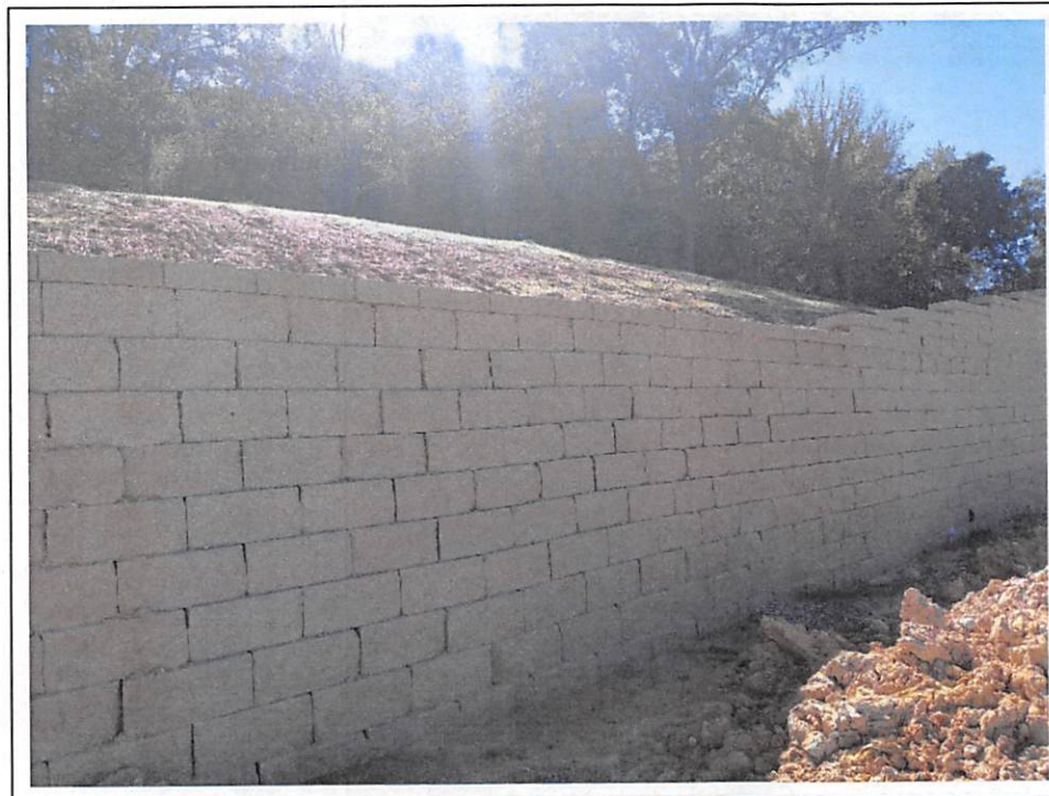
Photo #2: Looking east at Wall #1. Seed and straw are in place behind the wall.
