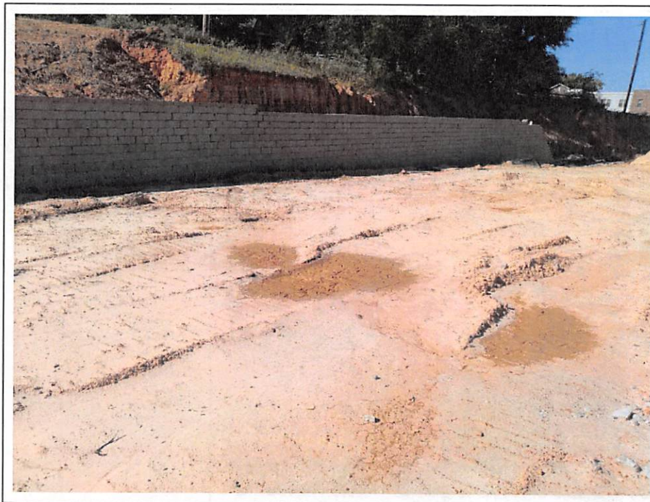
Photo #4: Wall #1 looking south. Final grading and seed/straw are needed behind the wall
