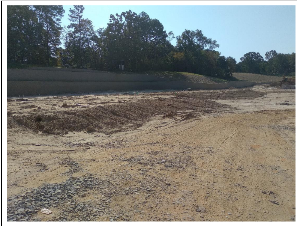
Photo #3: Wall #1, #4 and #5 looking southeast
