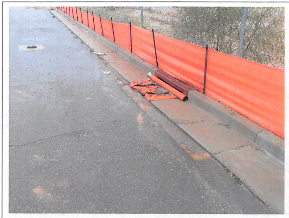
Photo #7: Curb inlet silt bag in good repair and functional,
