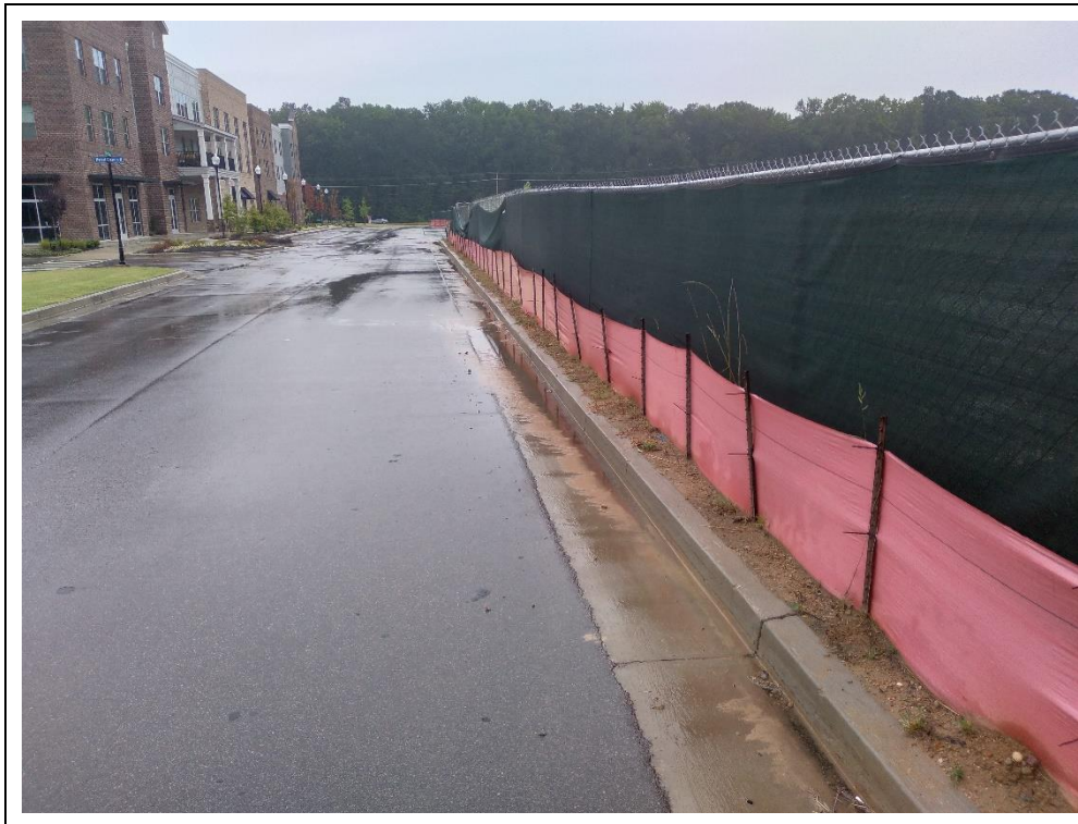
Photo #4: Silt fence in good condition along Village Market Lane looking north
