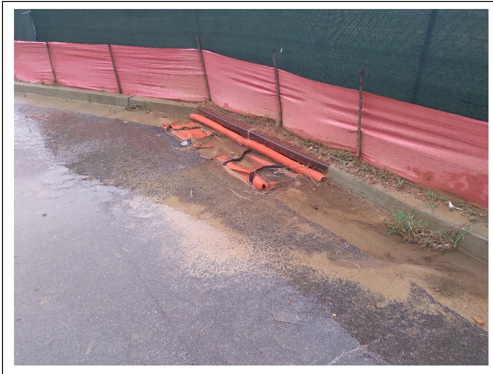
Photo #5: Inlet protection along Village Market Lane looking east
