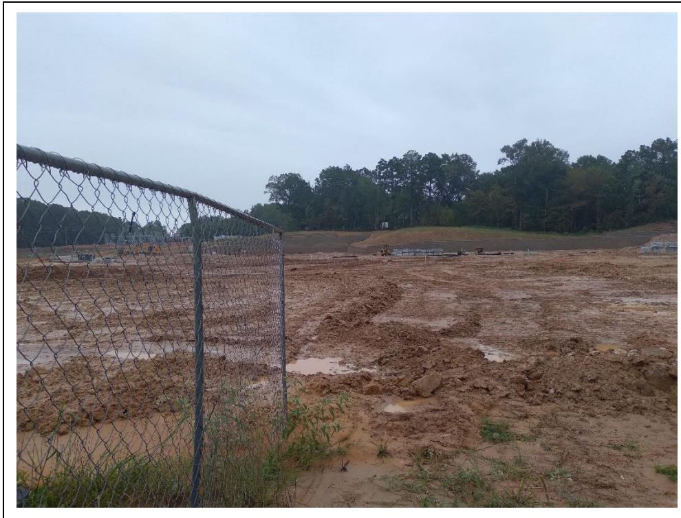
Photo #3: General site looking east
