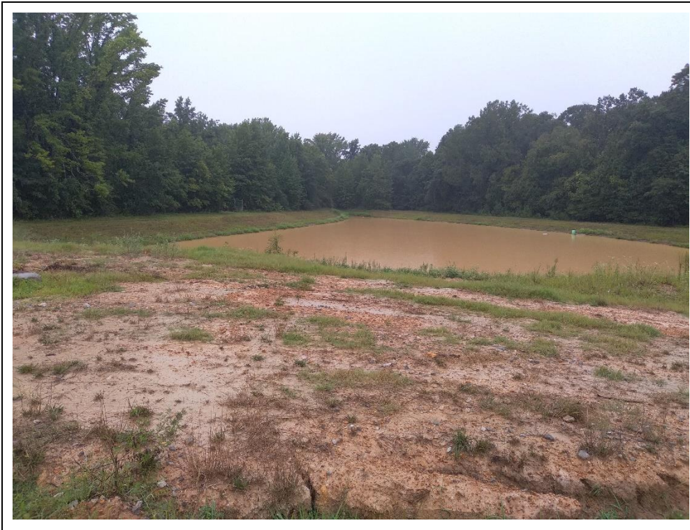
Photo #1: Detention Pond looking west. Cloudy conditions are due to rain overnight and earlier in the day
