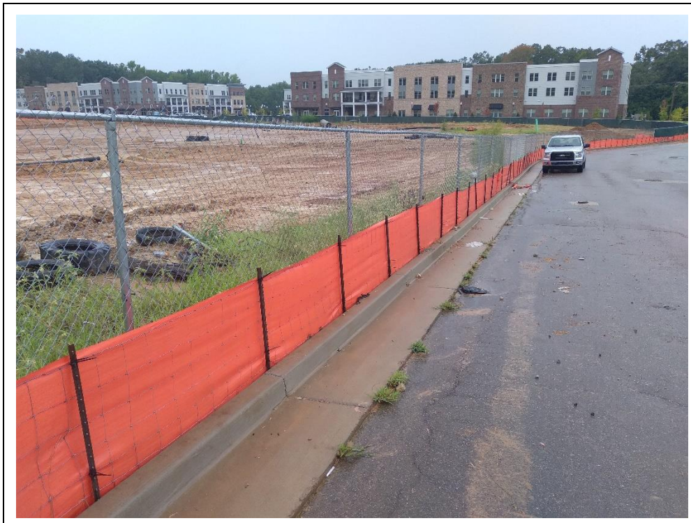
Photo #6: Silt fence along Shady Village Lane looking south
