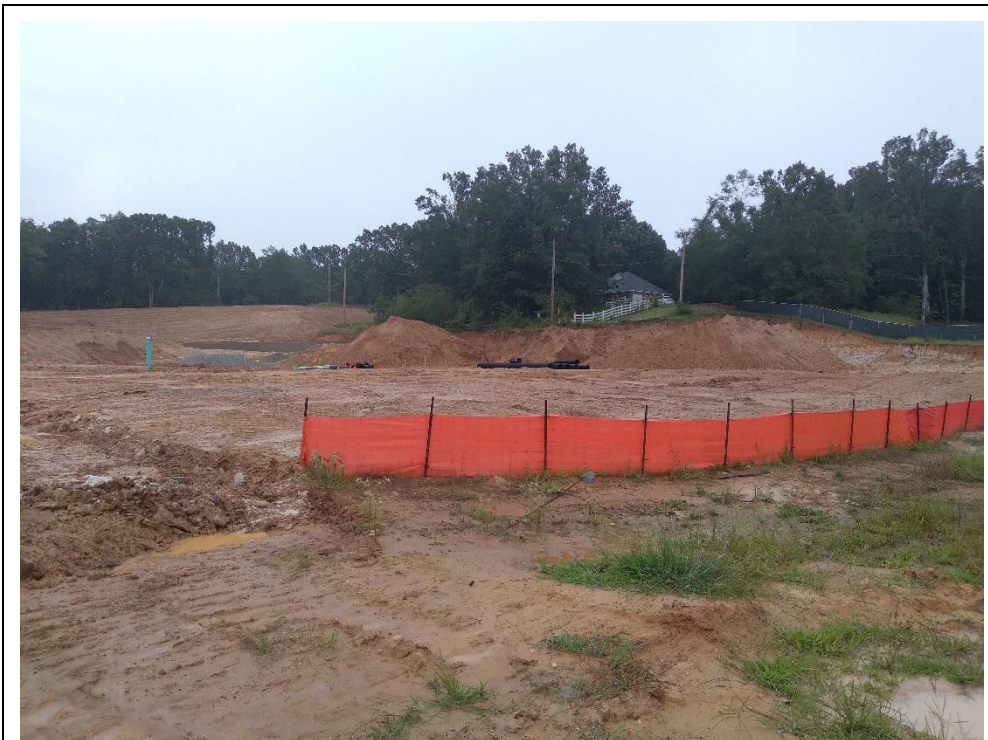
Photo #2: Looking east from Village Market Lane. Underground utilities are incomplete at the south end.
