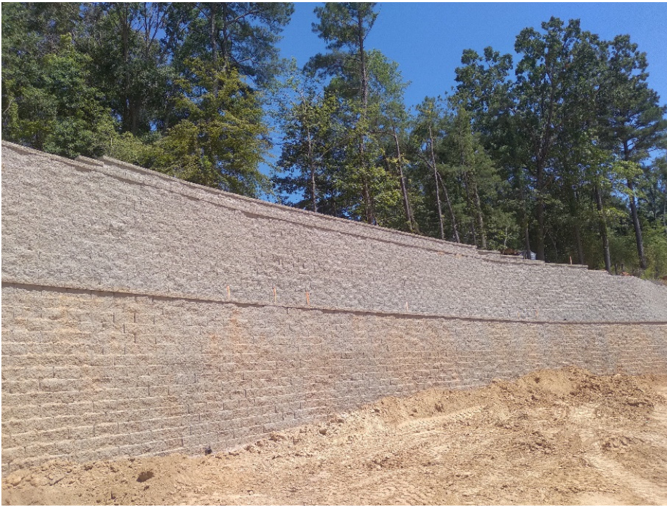
Photo #5: Walls #1, #4 and #5 looking east
