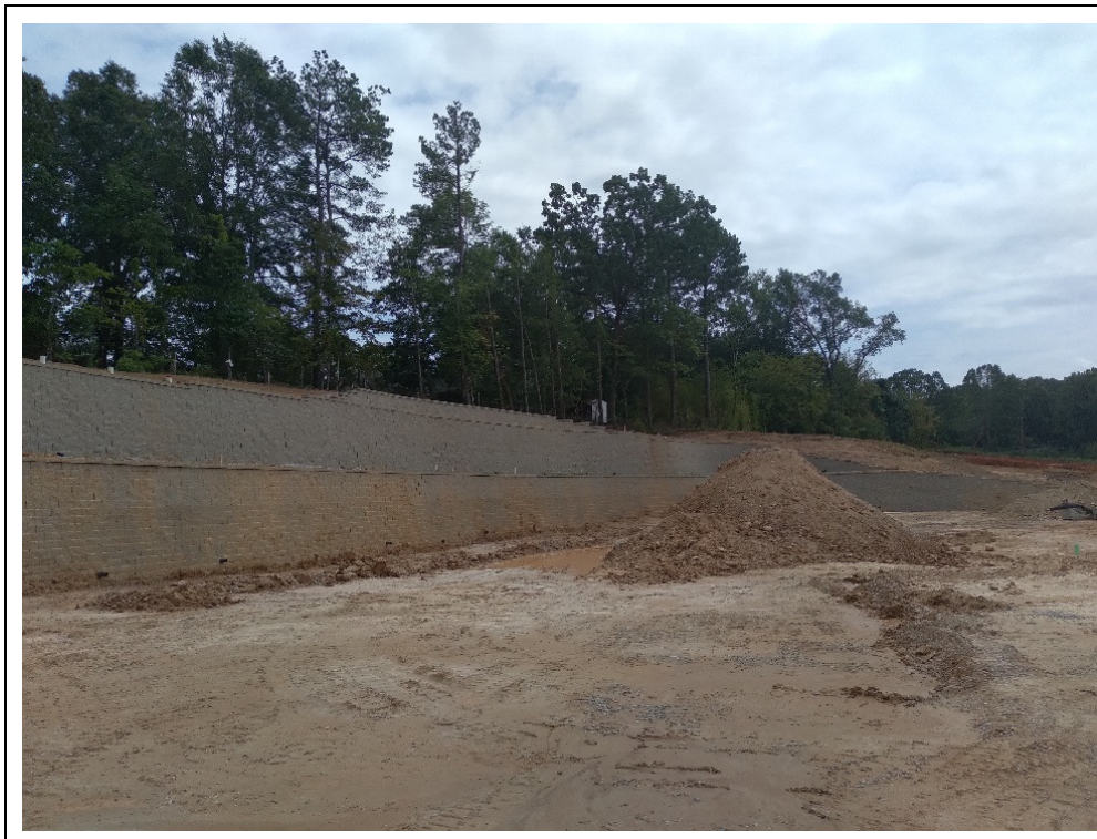
Photo #4: Wall #1 & #4 looking south
