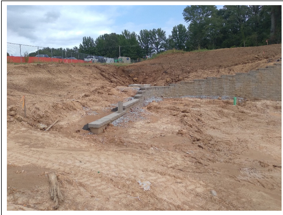
Photo #3: Wall #1 looking east
