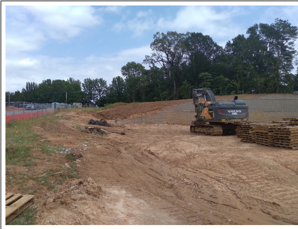
Photo #1: Looking east from entry gate.
