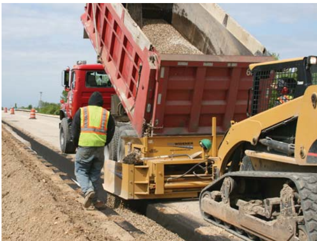
Trench backfilling with the FH Model.
