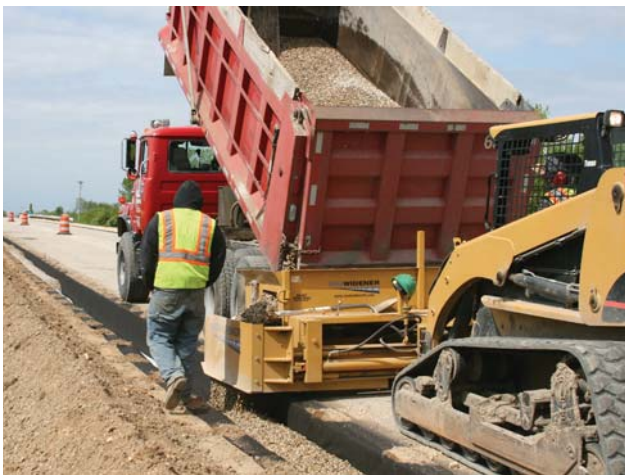
Trench backfilling with the FH Model.
