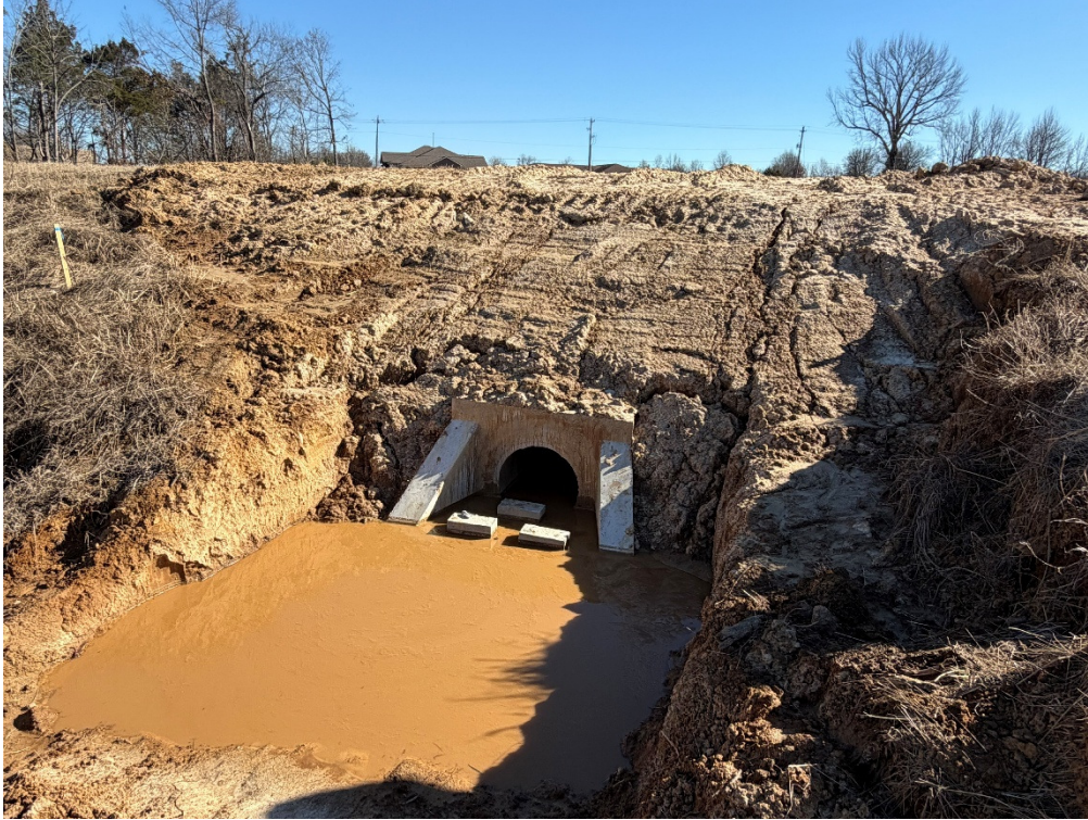
Photo 3: Storm drainage that has been installed.
