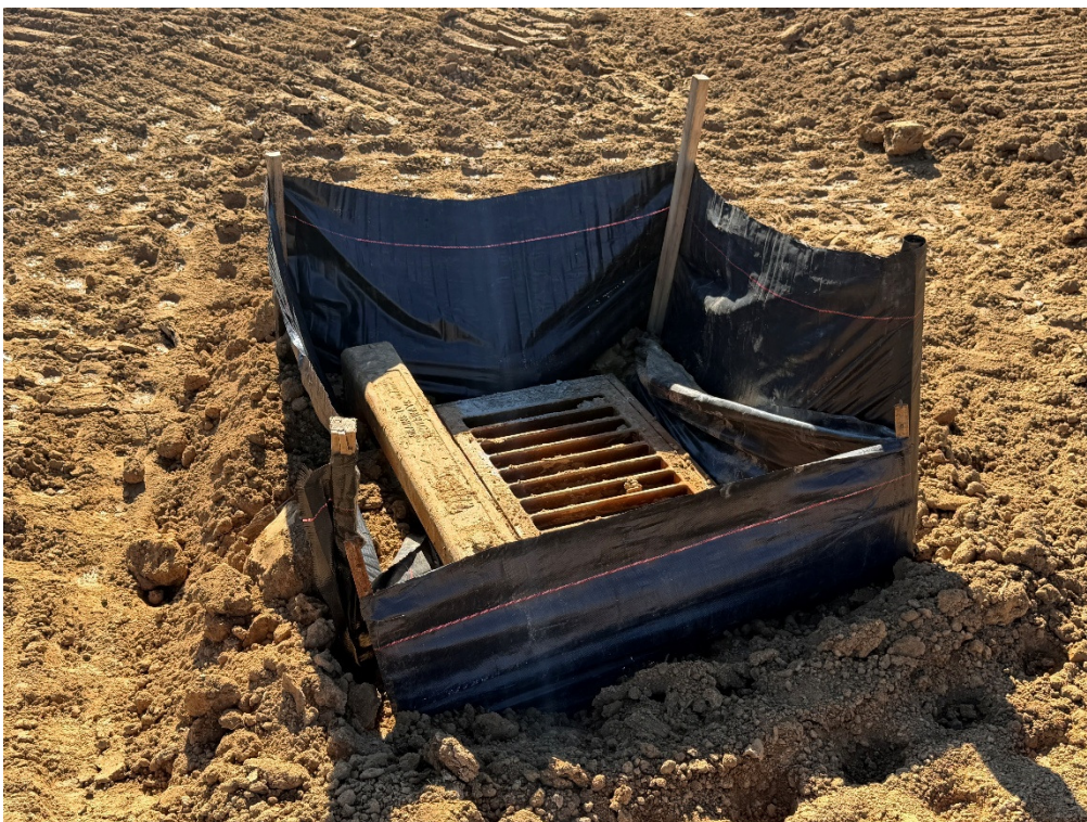
Photo 6: Curb inlet that has been installed.
