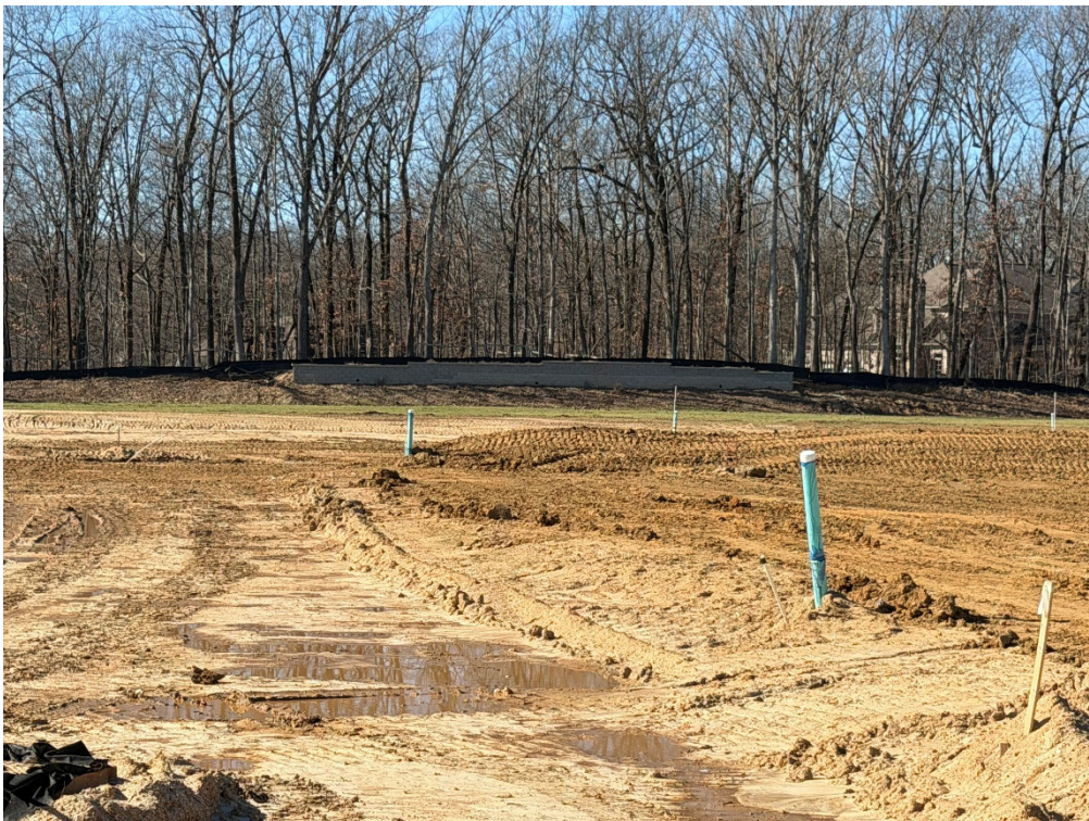
Photo 4: Sanitary Sewer service lines that have been stubbed up at lot locations.
