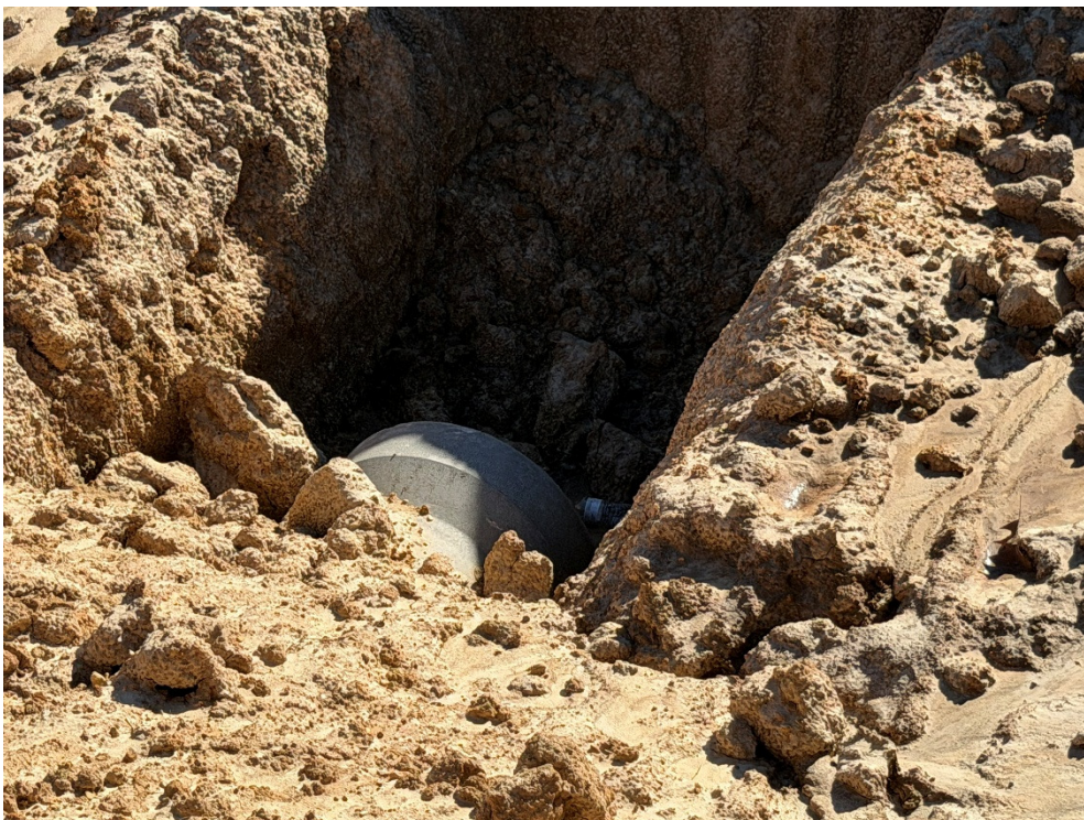
Photo 2: Storm Drainage in process of installation.
