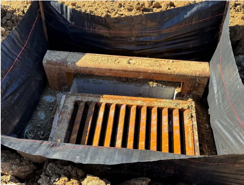
Photo 7: Curb inlet that has been installed.
