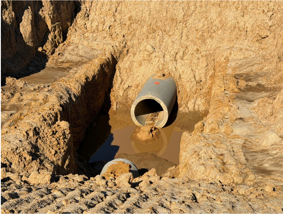
Photo 1: Storm Drainage in process of installation.
