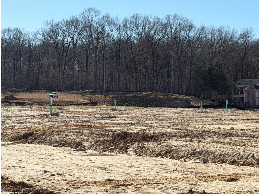
Photo 5: Sanitary Sewer service lines that have been stubbed up at lot locations.
