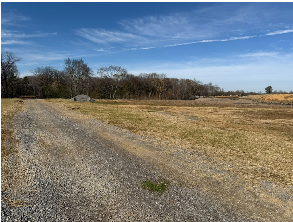
Photo 4: The slopes alongside the Lift Station Rd. have been temporarily seeded and mulched to prevent erosion.
