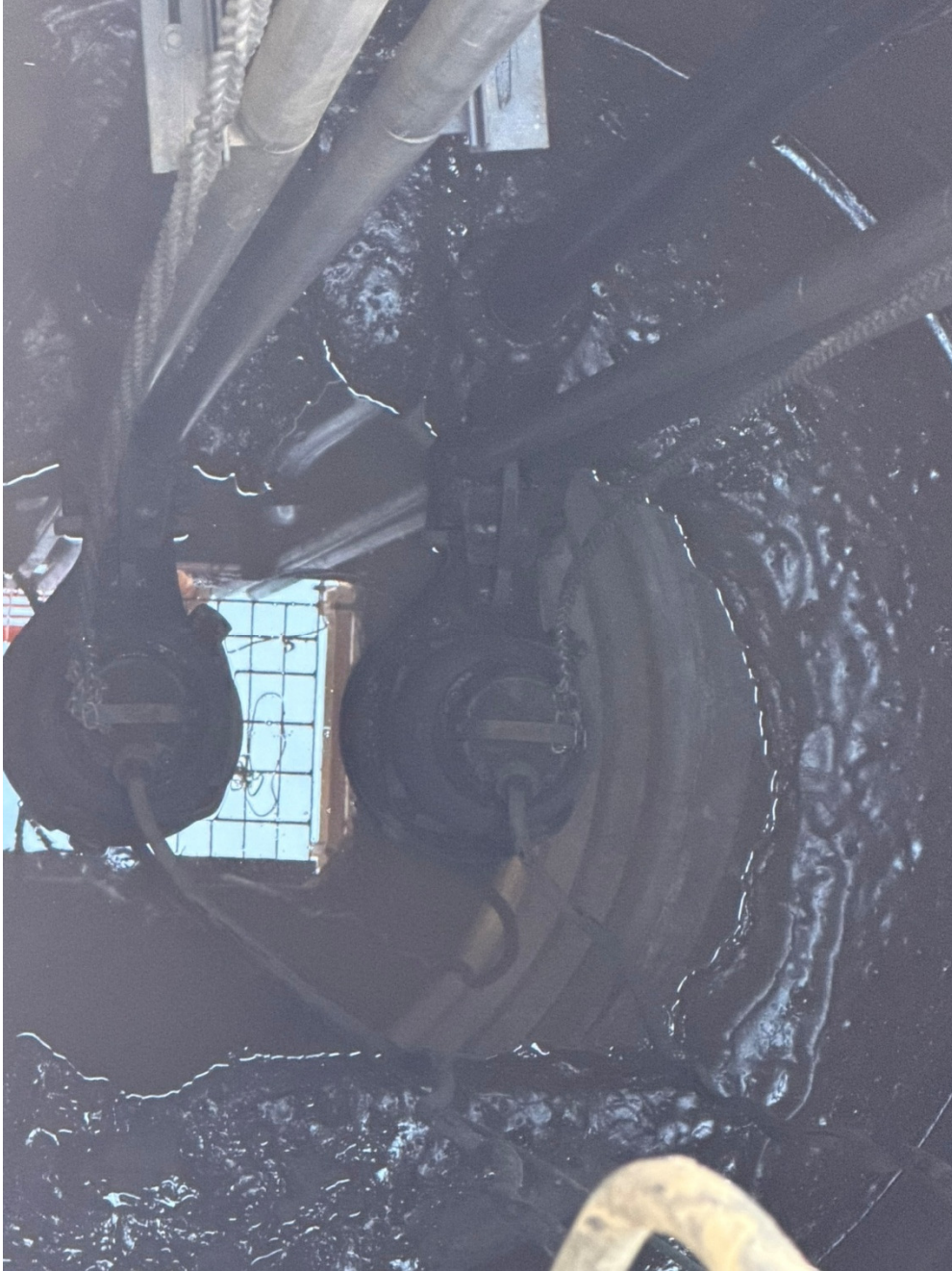
Photo 1: Pumps have been installed at the Lift Station.
