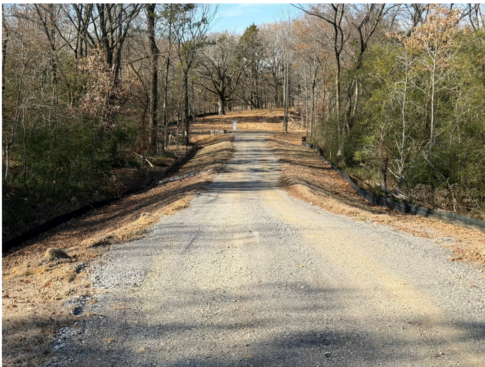
Photo 6: Additional Gravel has been used on the Lift Station Rd.
