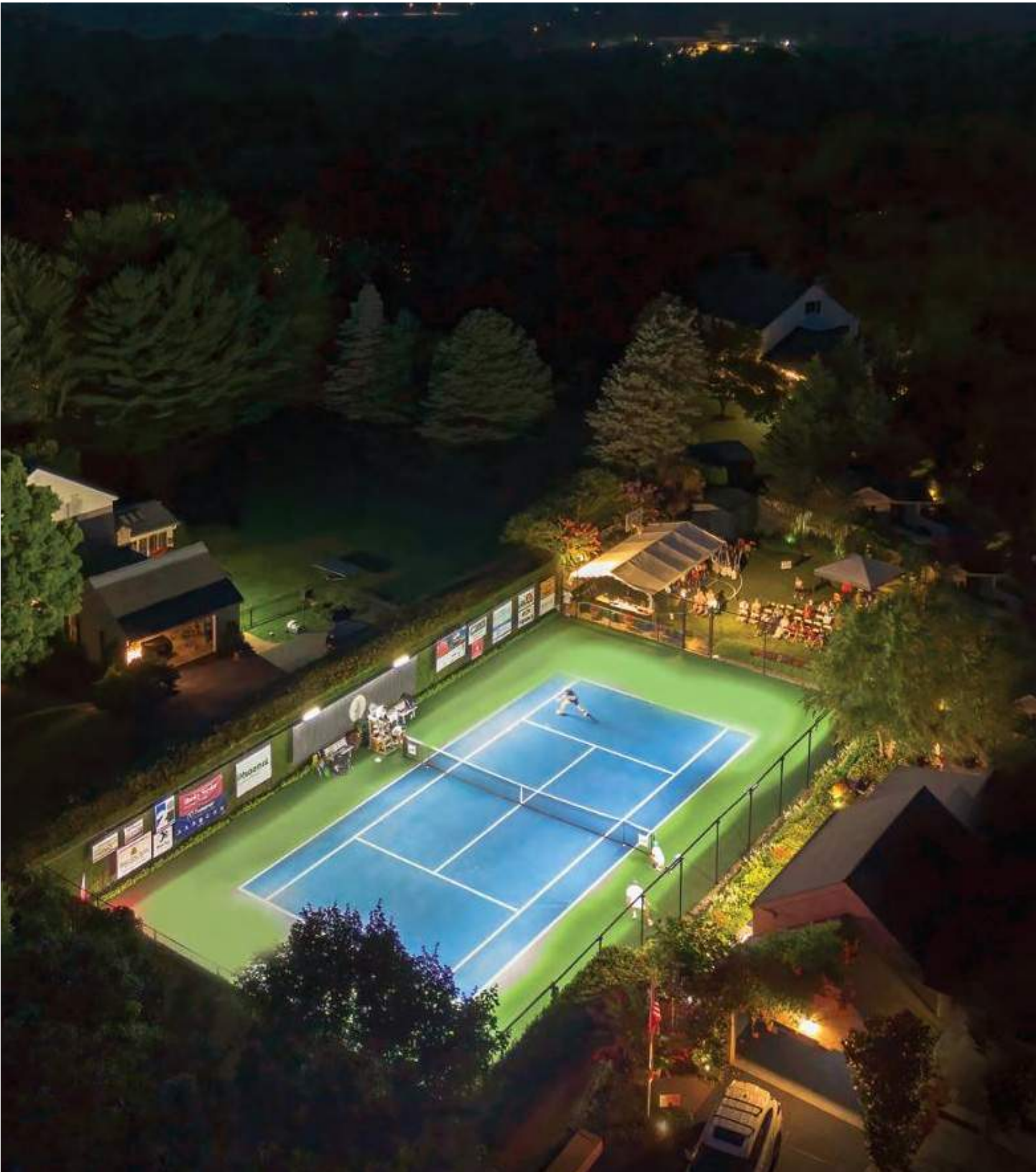
TENNIS COURT LIGHTING
