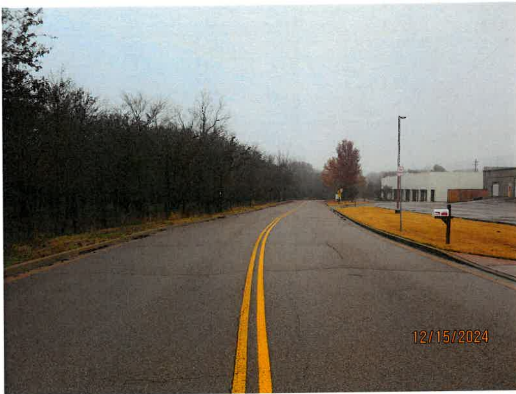
Typical street scene – looking east along Huff n Puff Road – subject property on left
