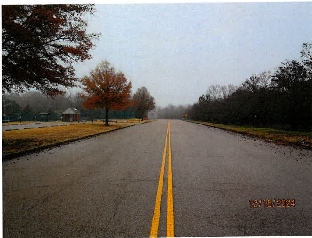
Typical street scene – looking east along Beverle Rivera Drive – subject property on right – photo taken at west end of site
