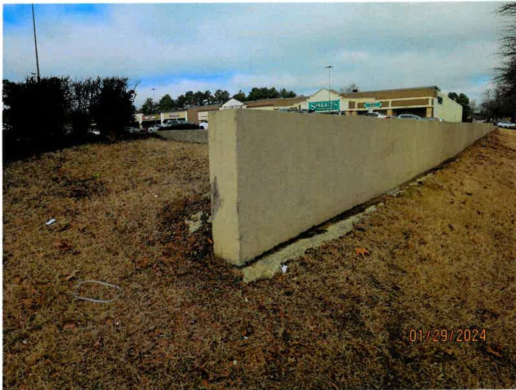
Improvement No. 2 – tall retaining wall
