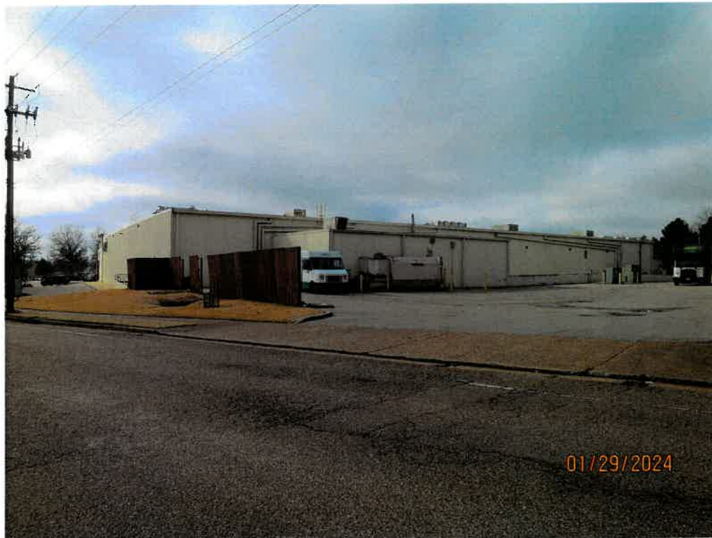
Larger parcel – looking southwest from northeast corner
