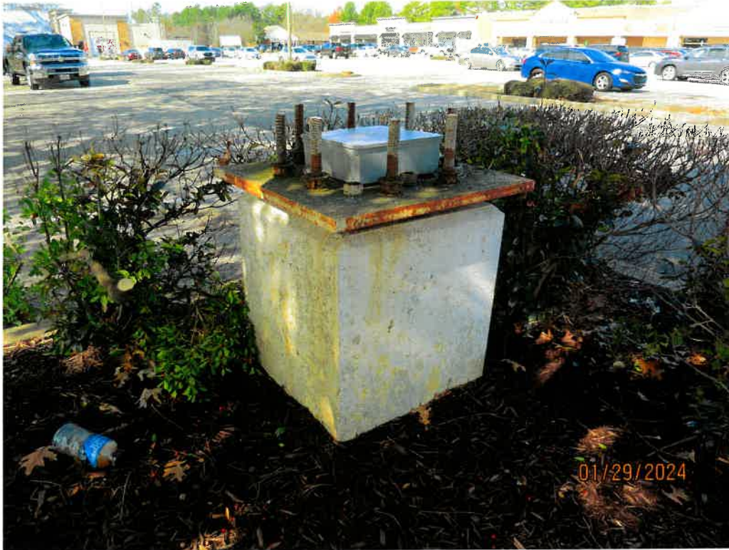
Older concrete sign base in permanent sewer easement area
