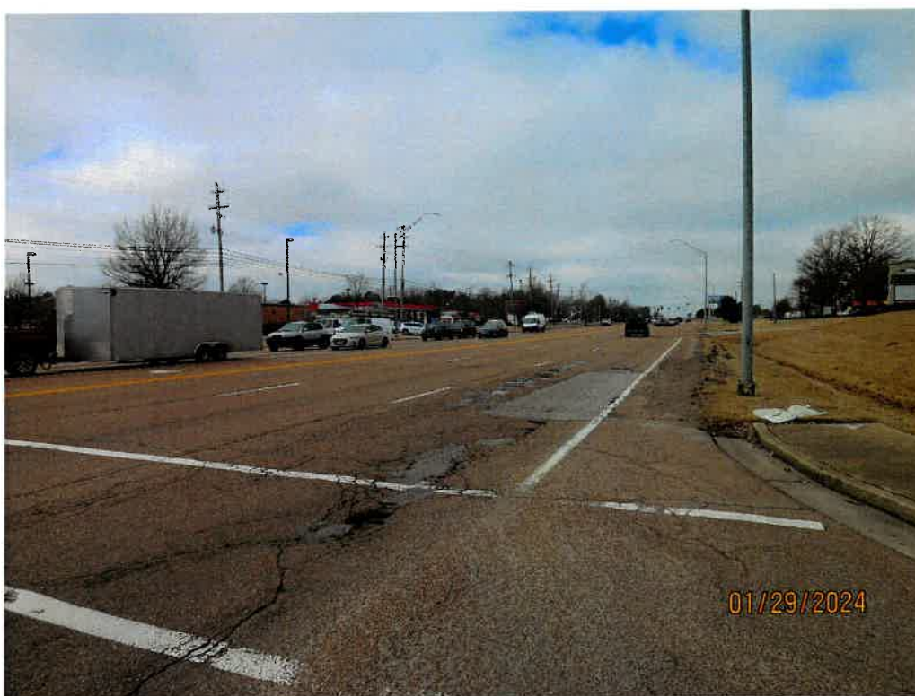
Typical street scene – looking west along Highway 64 – subject property on right
