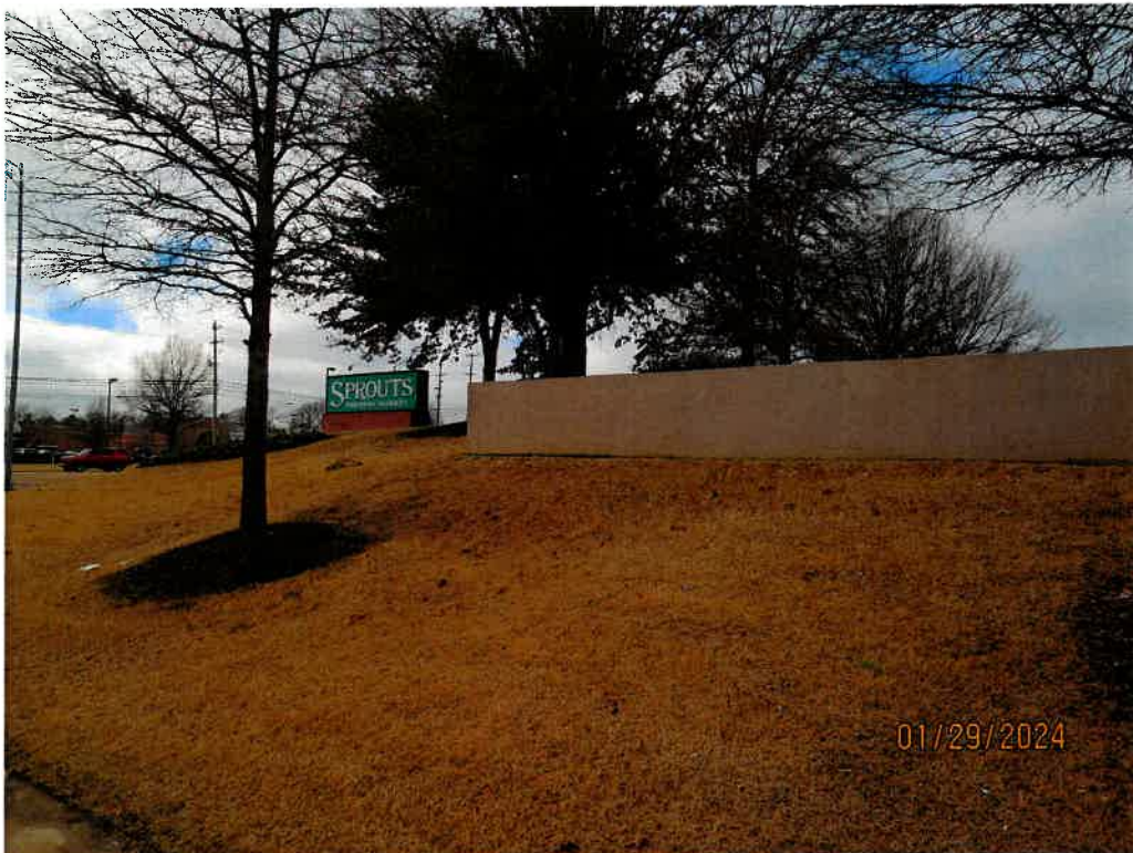
Permanent sewer easement area – looking southwest
