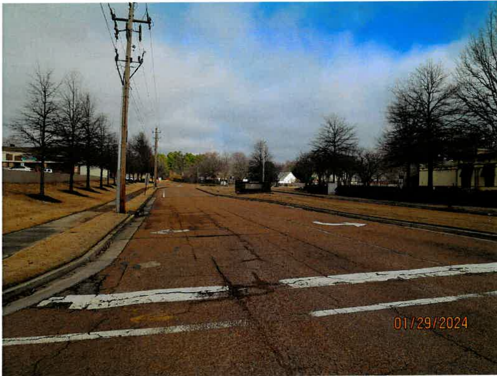
Typical street scene – looking north along Fletcher Trace Parkway – subject property on left
