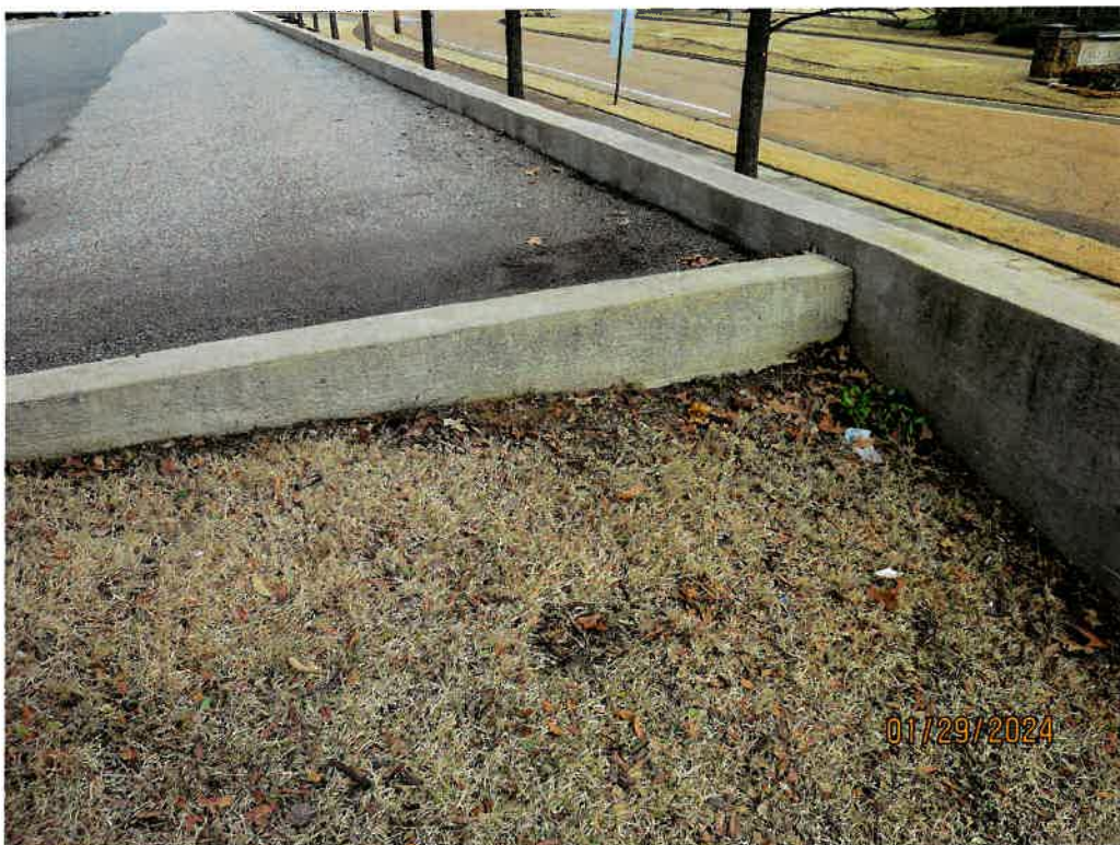
Improvement No. 2 – short retaining wall
