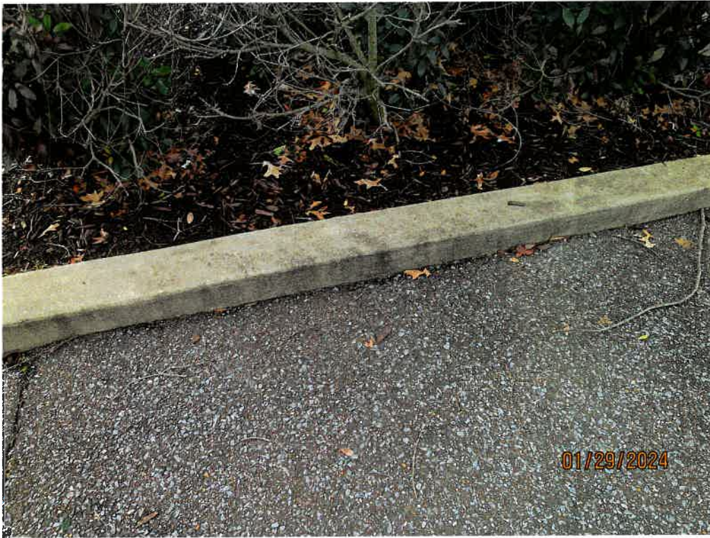
Improvement No. 3 – poured concrete curbing
