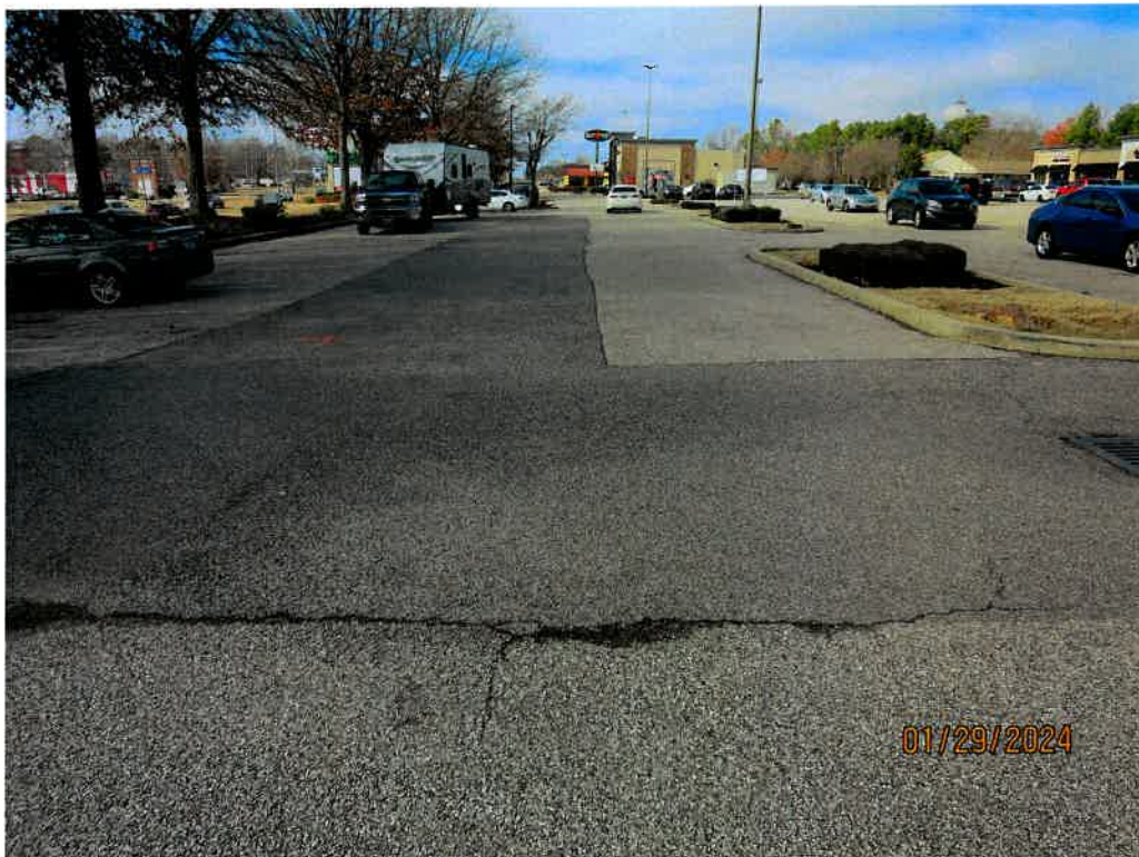
Temporary construction easement area – looking west from retaining wall
