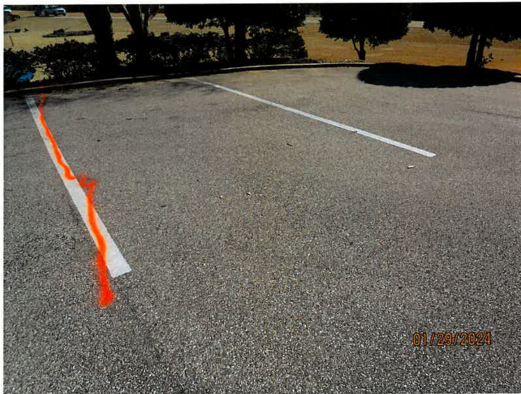
Improvement No. 3 – paved asphalt in sewer easement acquisition area
