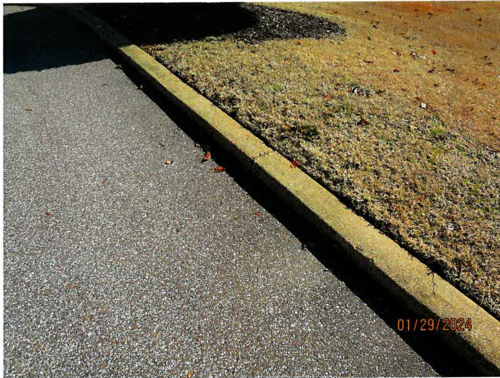
Improvement No. 2 – poured concrete curbing in sewer easement acquisition area
