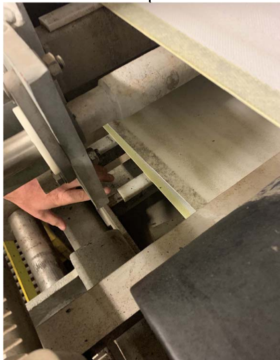
Wear strips worn
