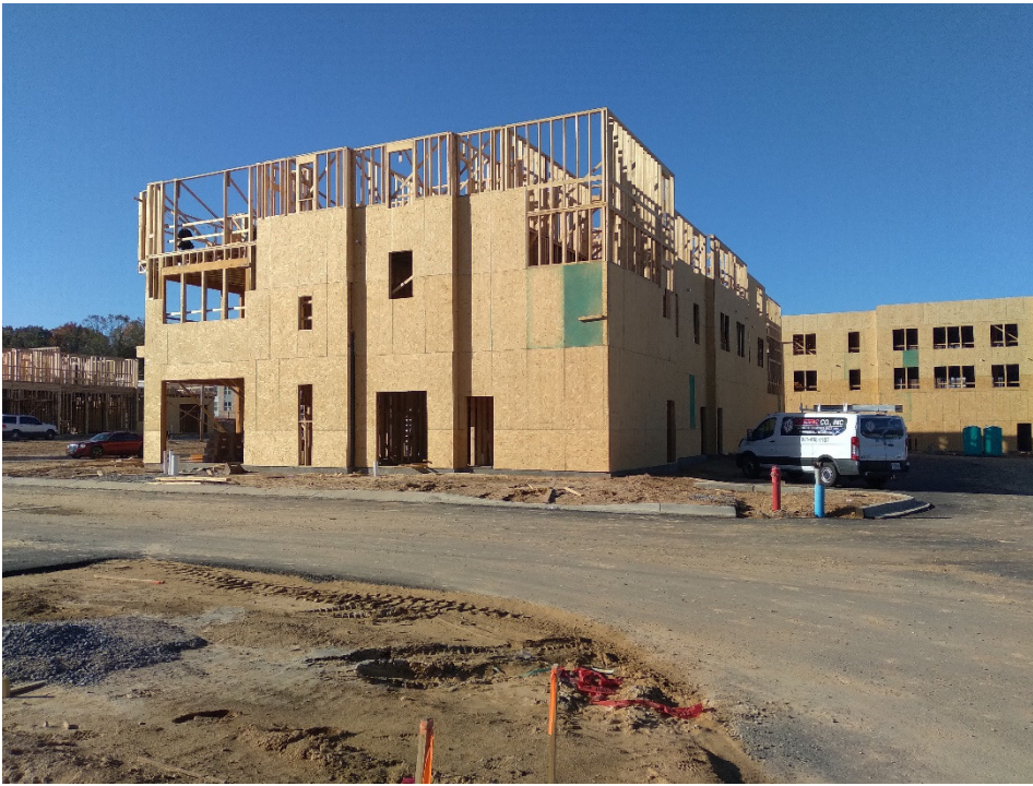
Photo #5: Asphalt base course has been installed at the north end of the site
