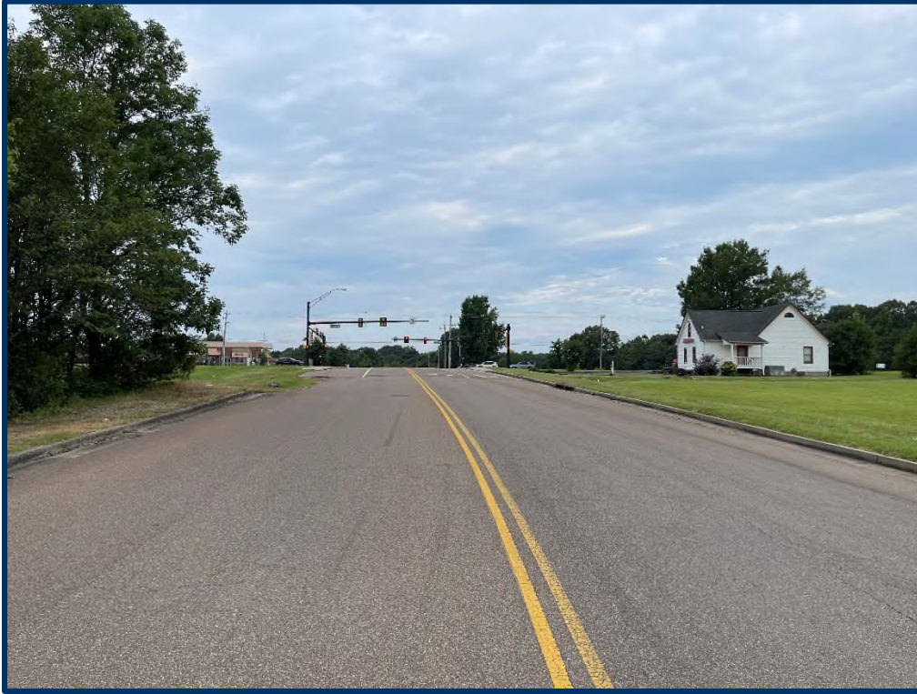
Looking southwest along Beverle Rivera Drive from Skyway Drive
